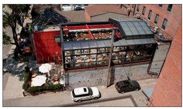
Energy efficient through natural ventilation With the roof open, heat rises and escapes. Mechanical air conditioning and dehumidification are not required. When the roof is closed, thermal breaks and vapor barriers control condensation and air filtration. The solar gain offsets much of winter heating requirements, all of which adds up to energy savings of up to 27% over traditional construction.
