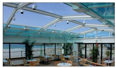
Maintenance free Unlike steel framing, OpenAire's maintenance free, thermally broken aluminum framing system stands up to moist, chemical atmospheres, in any climatic region.
