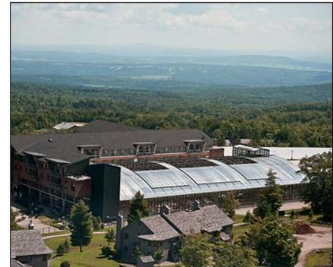
**6 Maintenance free** Unlike steel framing, OpenAire's maintenance-free, thermally broken aluminum framing system stands up to moist, chemical aquatic atmospheres and never needs to be repainted.
