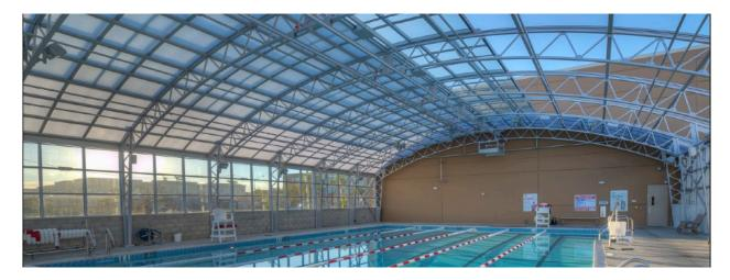
have led to the sudden collapse of ceilings, along with deaths and injuries. The cause was chloride-induced stress corrosion cracking (SCC).<sup>7</sup>
