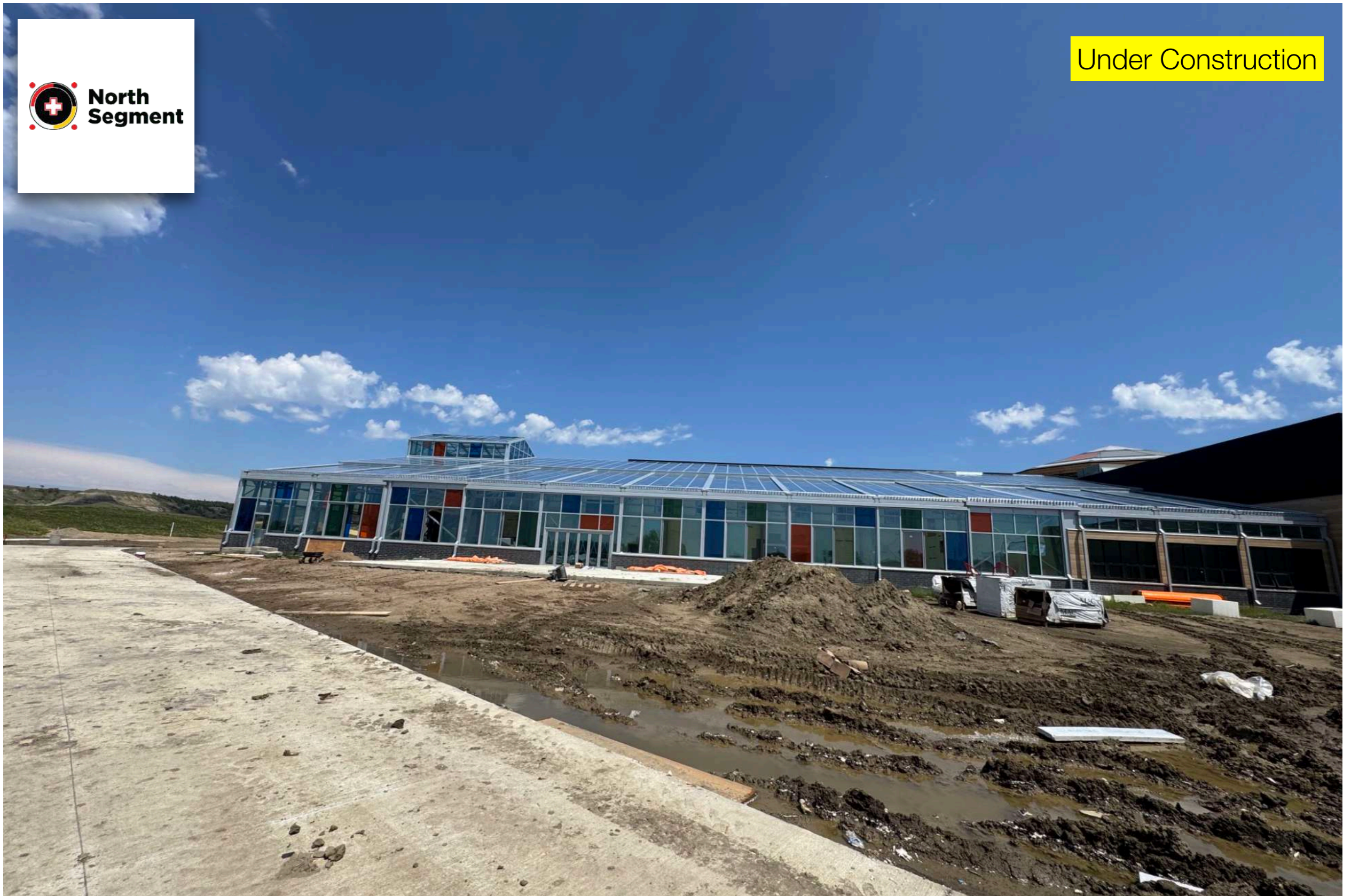
North Segment Community Center New Town, ND, USA
