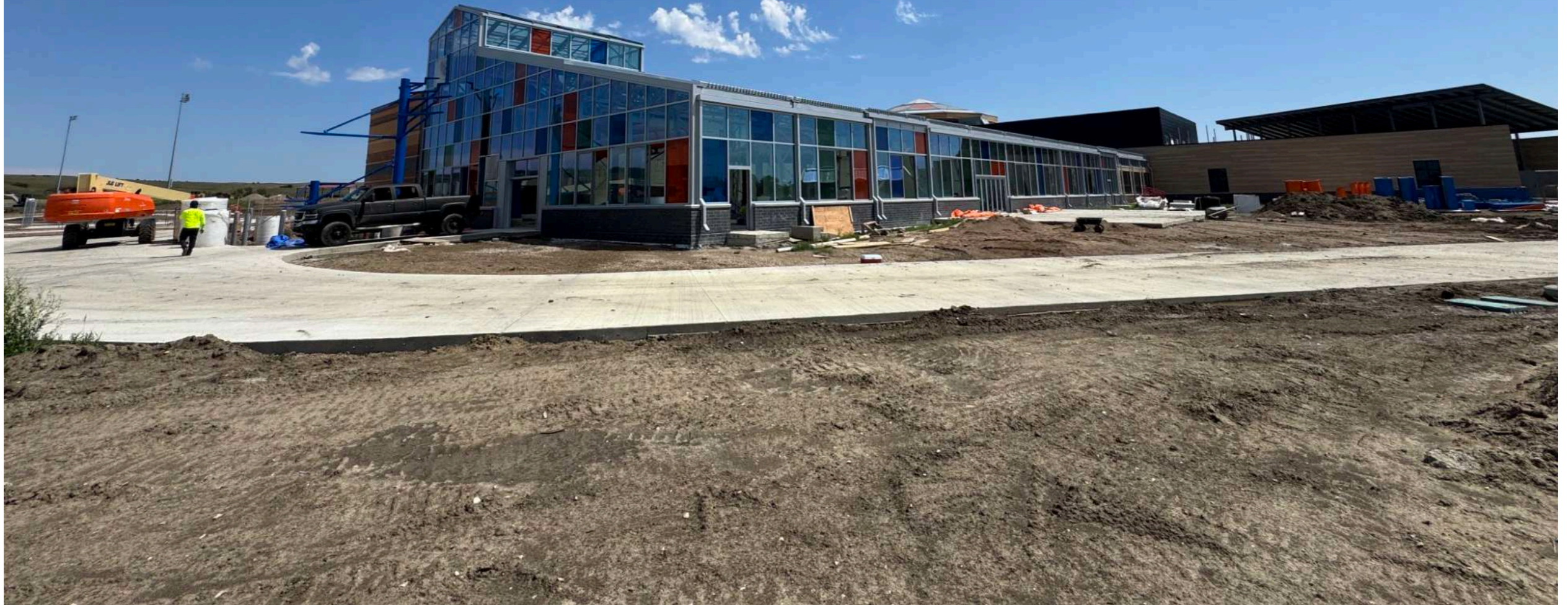
North Segment Community Center New Town, ND, USA
