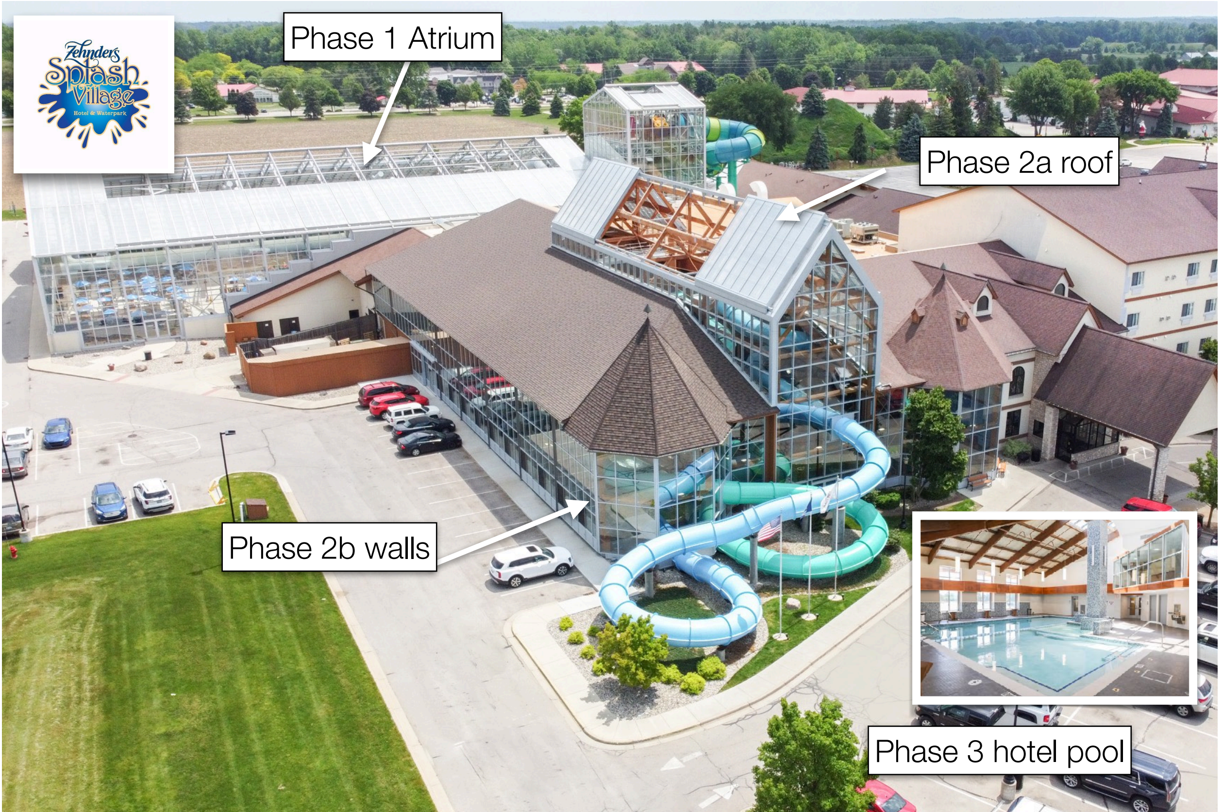
Zehnders Splash Village Waterpark Multi Phase Renovation Frankenmuth, MI
